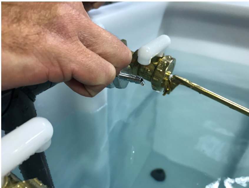
Default factory setting - a constant steady drip from the hand operated water dump frequency valve outlet
