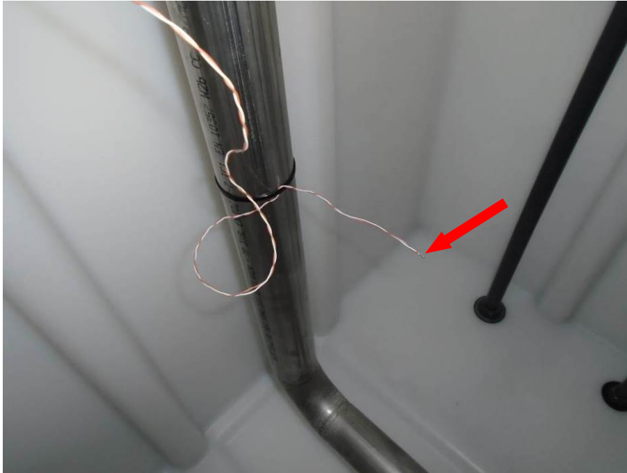
Figure 2.1.5 Additional middle thermocouple (installed by TÜV)
